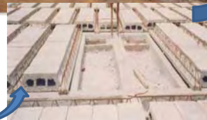
On site T Beams and Hollow block production for floor constructions
